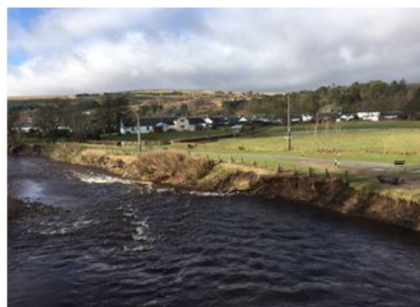
View of downstream right bank erosion from left hand bank
