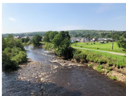
View of downstream right bank erosion from left hand bank
